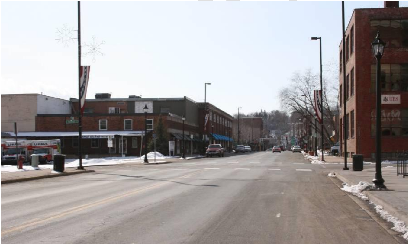
Figure 24. Existing Main Street at Mulberry Street
